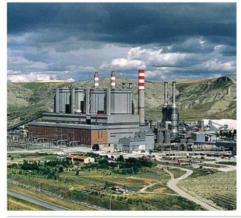
bistan plant in southeast Turkey (Figure 6). Unit A began operating in 1983 and Unit B in 2006. Unit A has attracted criticism as none of its flue stacks has a desulphurization unit, while its electrostatic precipitator system cannot handle the amounts of coal required when the plant is firing at full capacity. Furthermore, there is no fly ash dam facility at the plant, and the ash is stacked in an open dump, where it can be blown into surrounding areas by strong winds.
