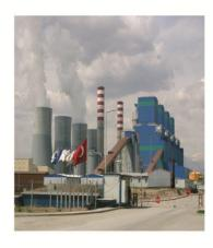
DOKAR has long been successfully sequestering the fly-ash a by-product of thermal power plant located eastern part of Turkey called "Afşin Elbistan". This is a coal fired plant powering up to 1.440MW. 4 units emitting immense amount of fly-ash forced us to compact & bury at 18 million cubic meter waste-dump-site which is designed by Dokar engineers using bulker-truck techniques.
